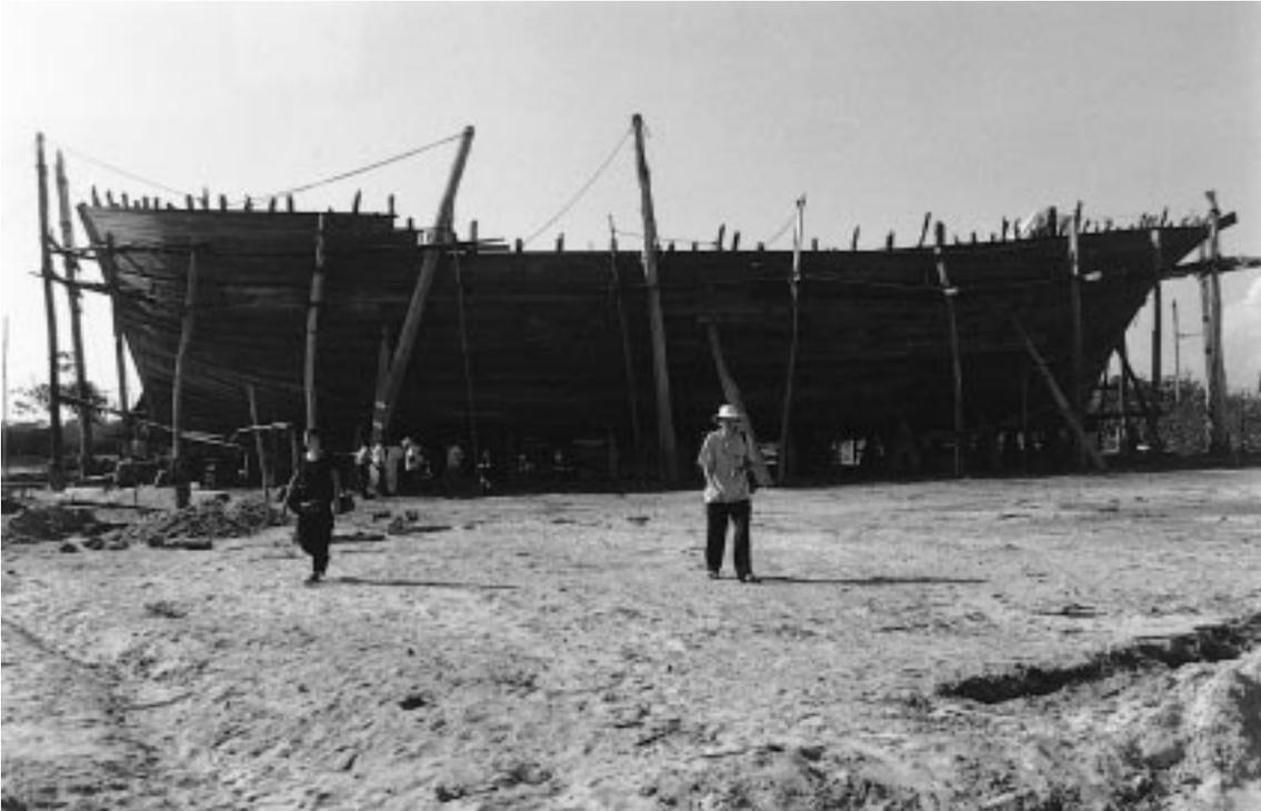
FIG. 2 – A *thoni* nearing completion on a foreshore building site at Tuticorin. Photo: S. McGrail
